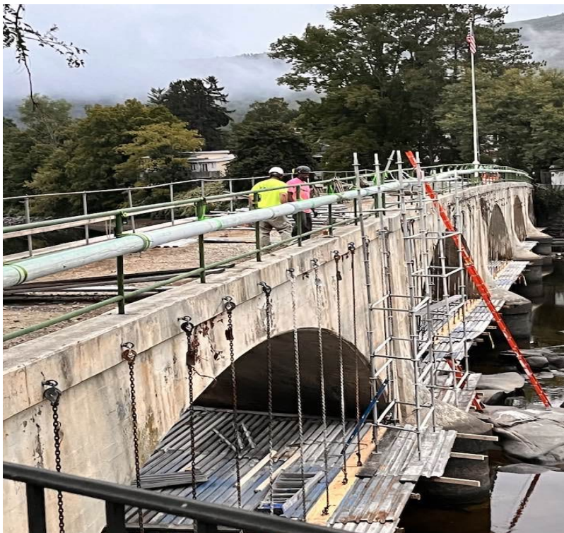
Shelburne Falls – Bridge of Flower being renovation to be completed 2025
